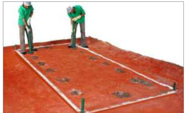
FIXING OF PEGS
